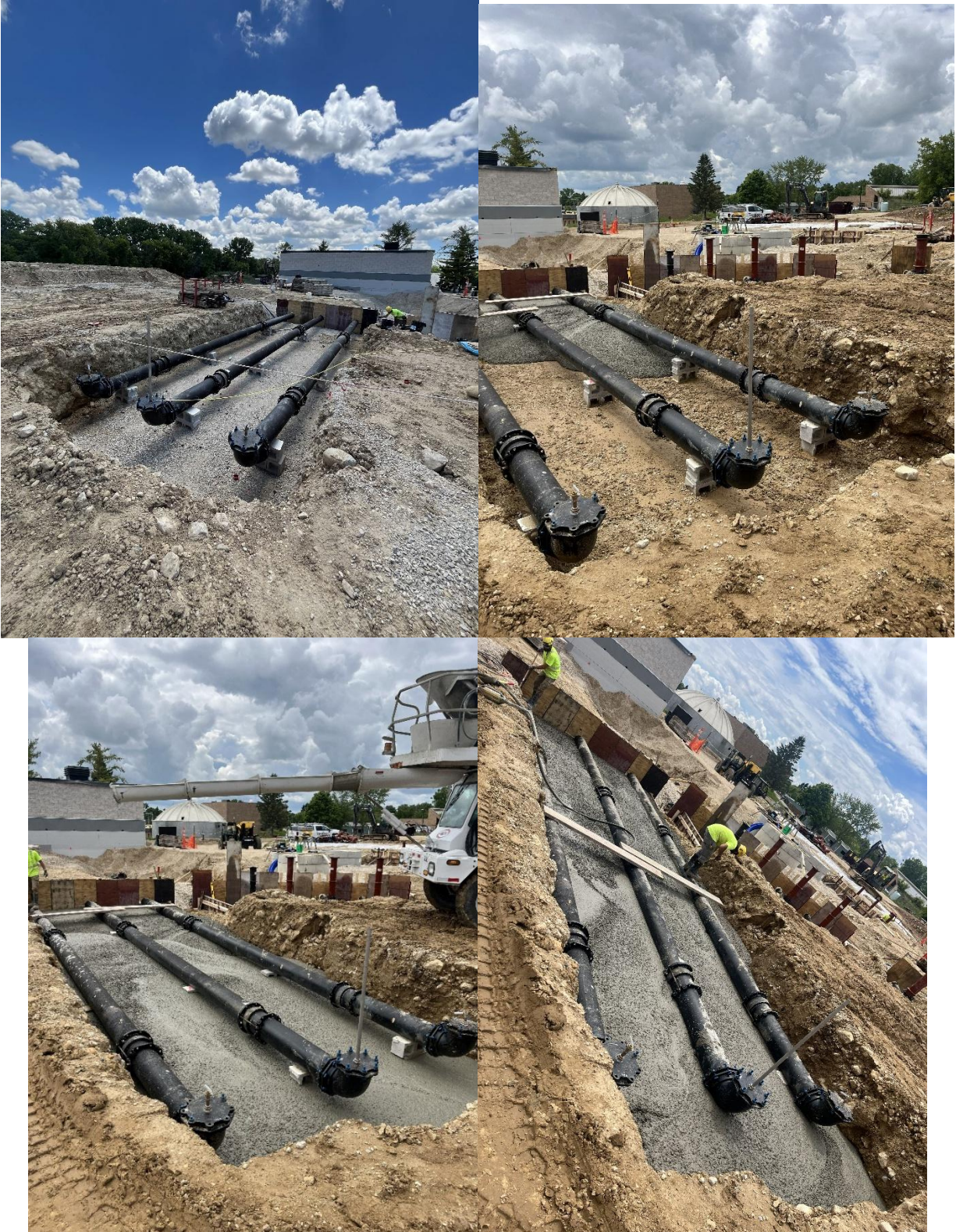
STR 600/700 Underground. Risers being installed and concrete encasements beginning to be poured.
