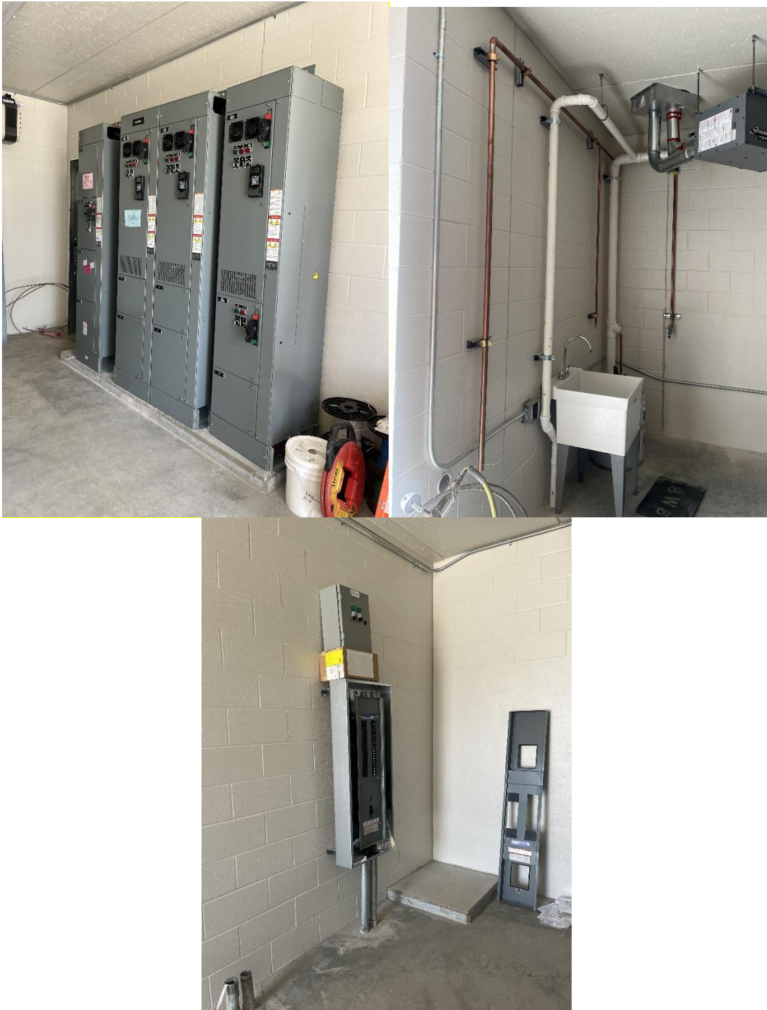
STR 650 and plumbing and electrical buildout.
