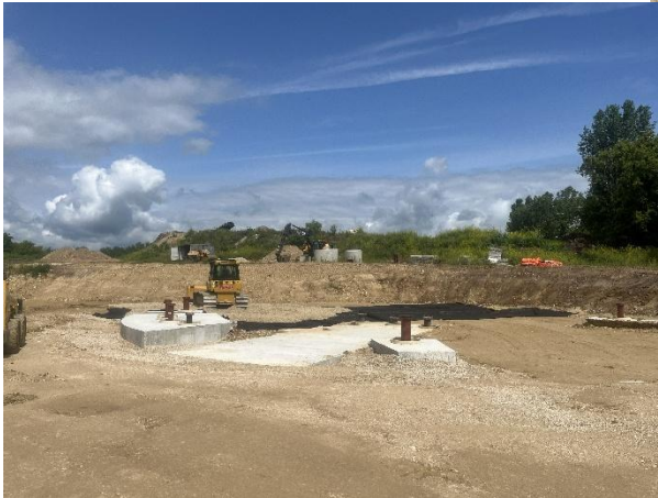
STR 600/700 concrete encasements and site grading/ graveling. Prep for DN tanks.
