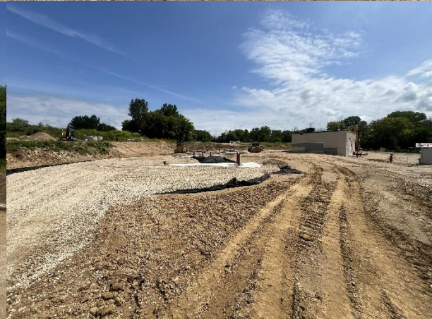
STR 600/700 concrete encasements and site grading/ graveling. Prep for DN tanks.
