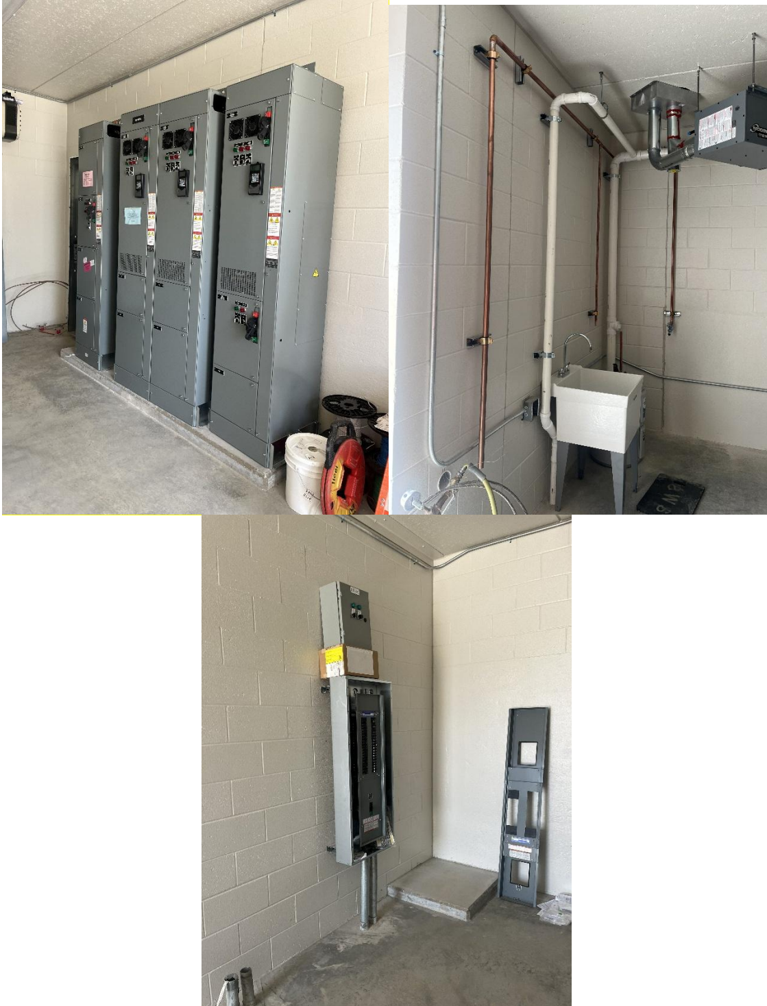
STR 650 and plumbing and electrical buildout.
