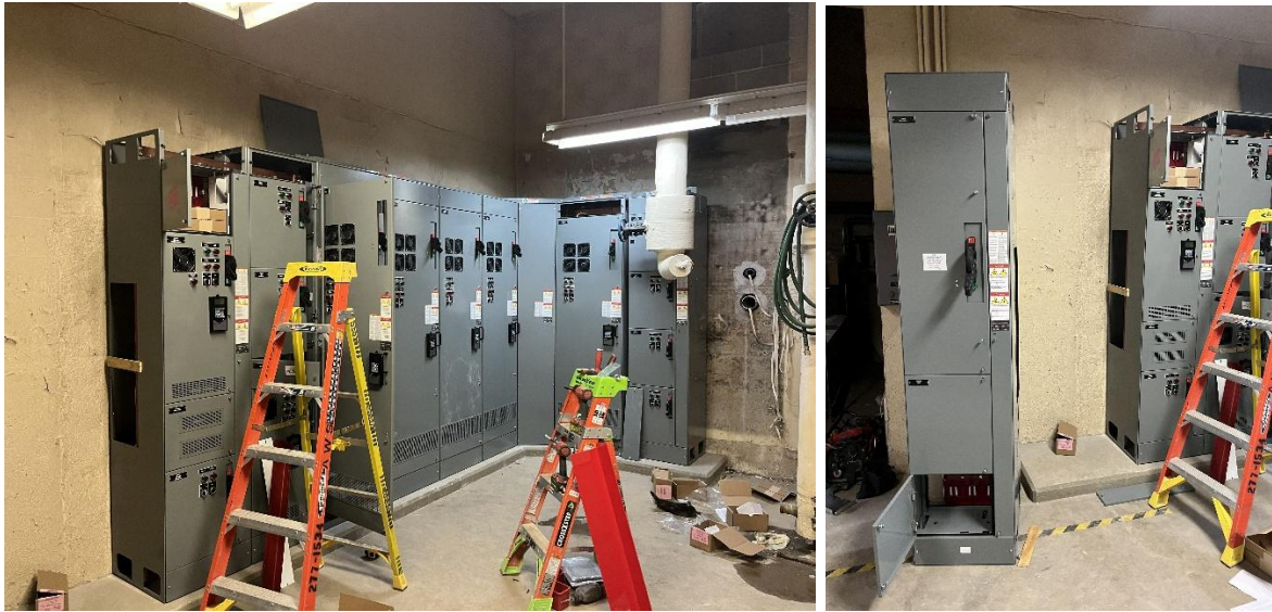
STR 100 East MCC Install.
