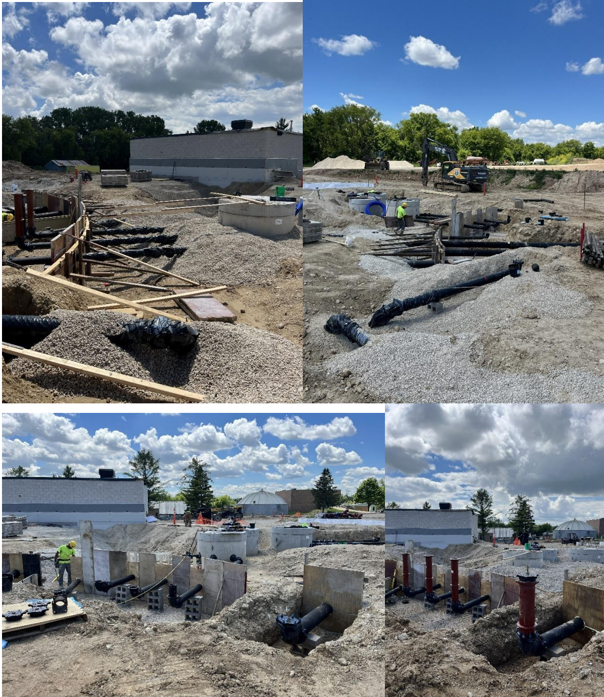
STR 600/700 Underground. Risers being installed and concrete encasements beginning to be poured.
