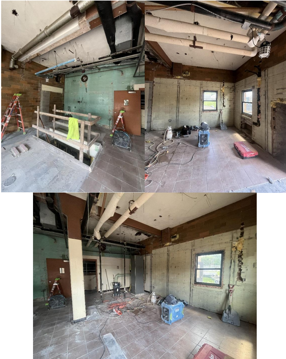
STR 100 area 4 demolition.
