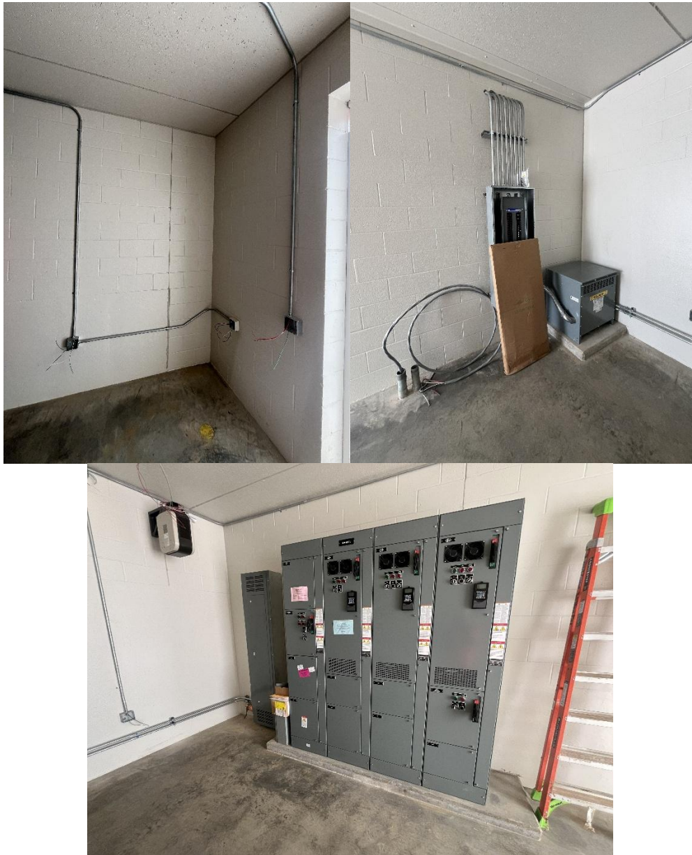
STR 650 electrical buildout continuing.
