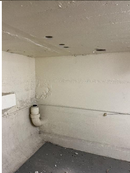
STR 100 area 4 demo and hatch prep (Say bye to Cold War Bunker).
