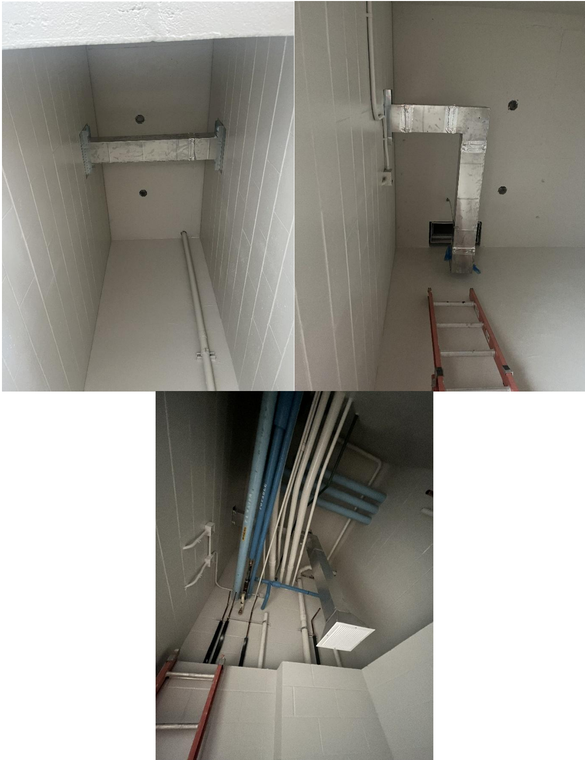
STR 100 Bathroom painting and HVAC.
