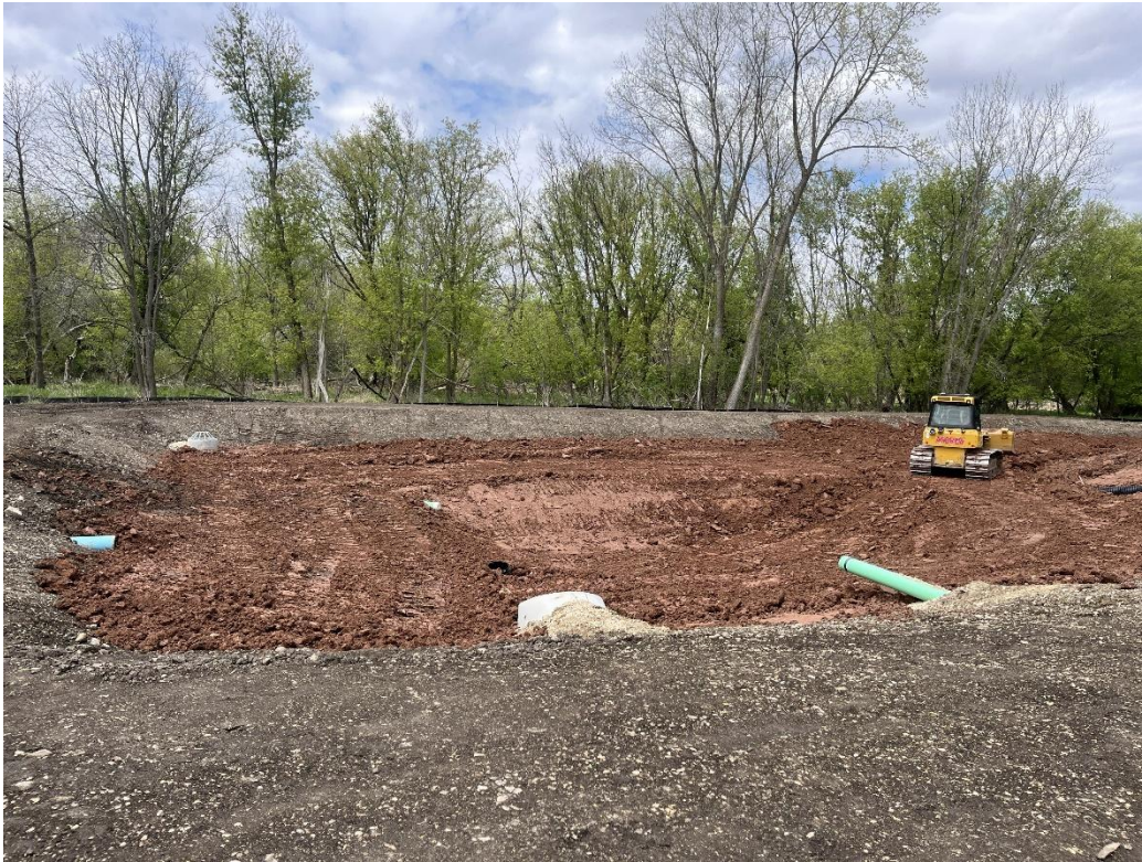
Clay liner going in West Wet Pond near STR 800.
