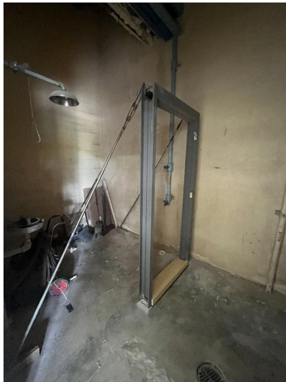
STR 100 bathroom wall beginning prep.
