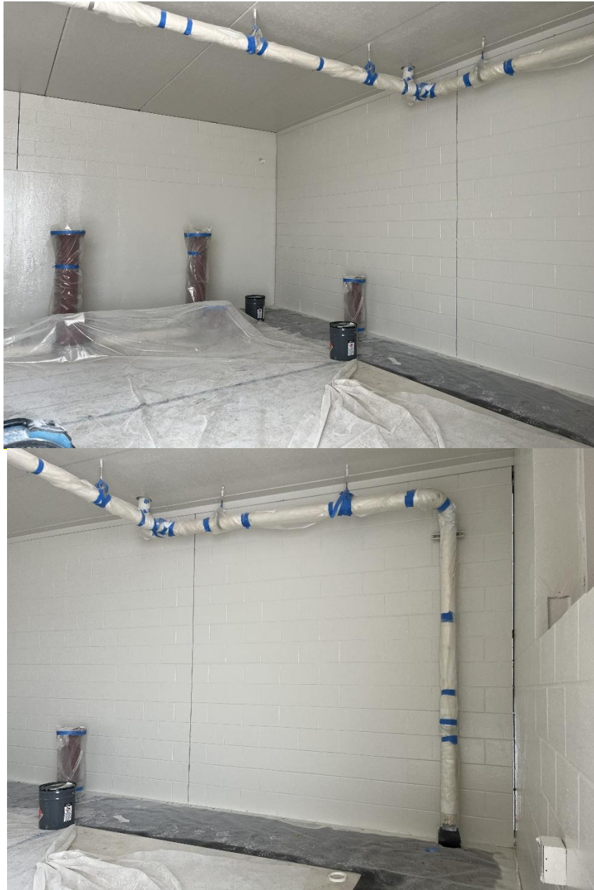
STR 650 Plumbing installed, painting being completed.
