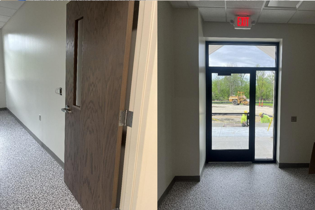
Doors and Door Hardware Installed in STR 800.
