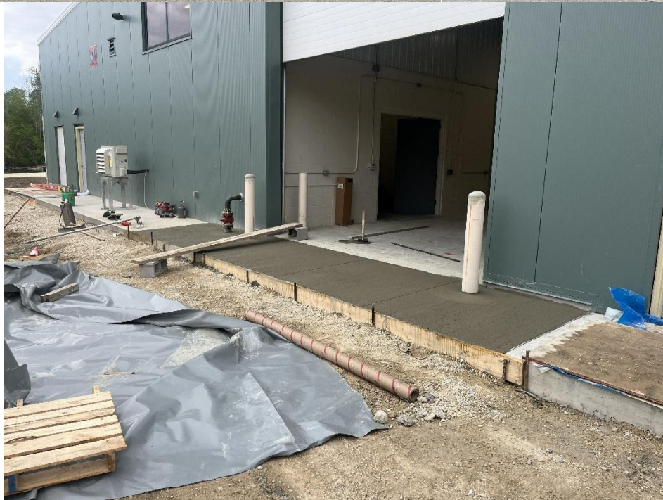
STR 800 / Site Concrete work continuing.
