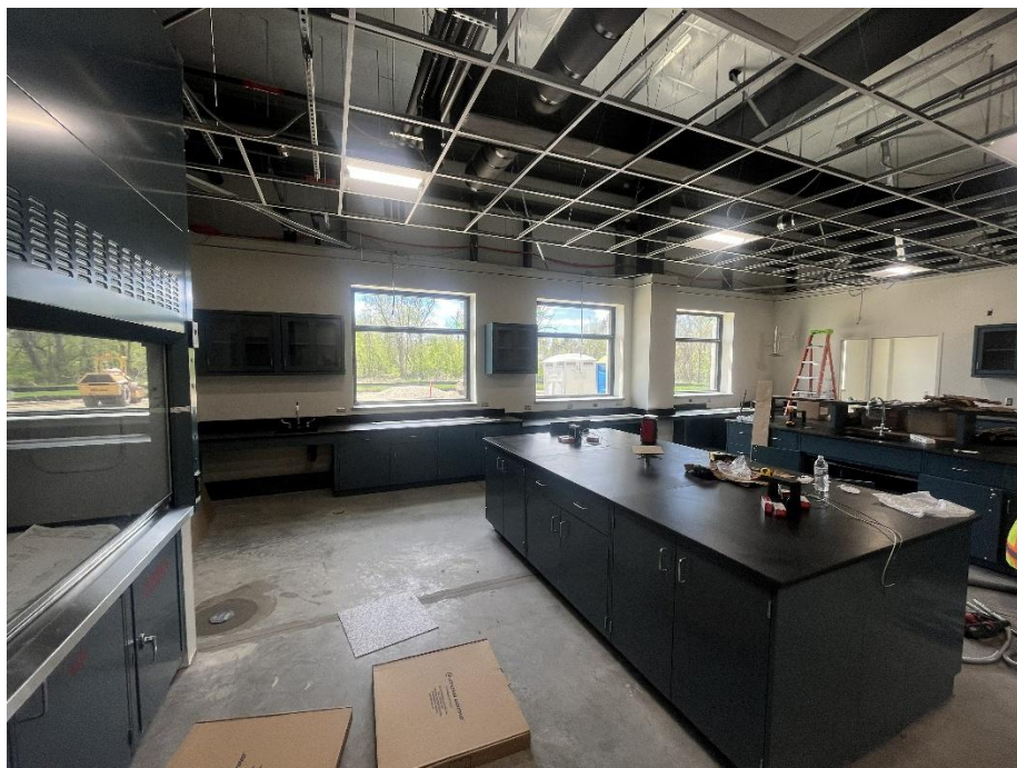
Laboratory casework installation complete.
