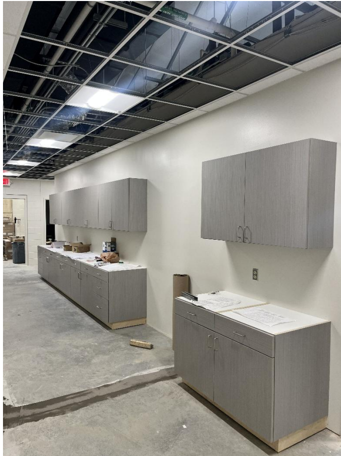
STR 800 hallway casework installed.
