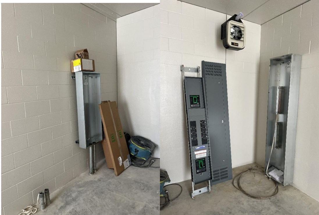
STR 650 electrical buildout beginning.
