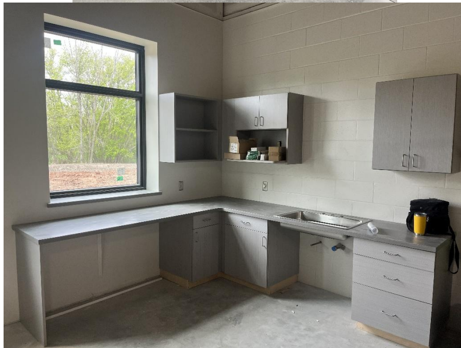
STR 800 team area casework installed. Break room casework in progress.
