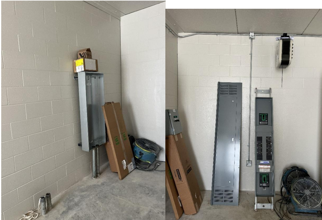
STR 650 electrical buildout continuing
