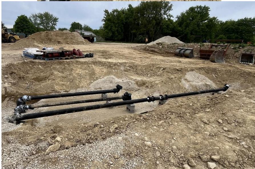
STR 650 underground piping and sludge manhole piping being installed.
