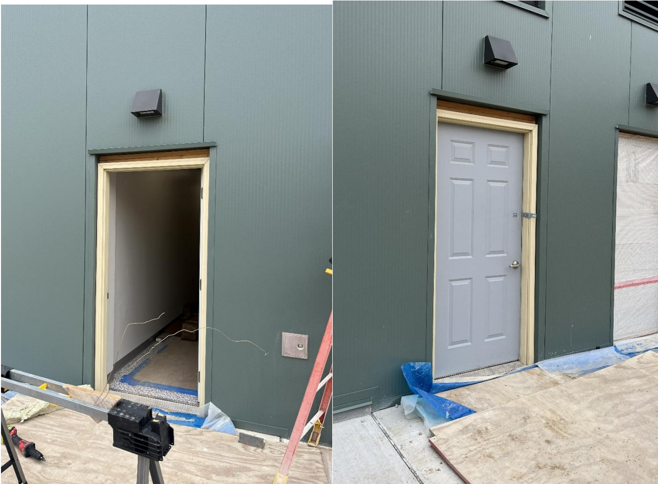
Exterior Doors and Door Frames being Installed in STR 800.
