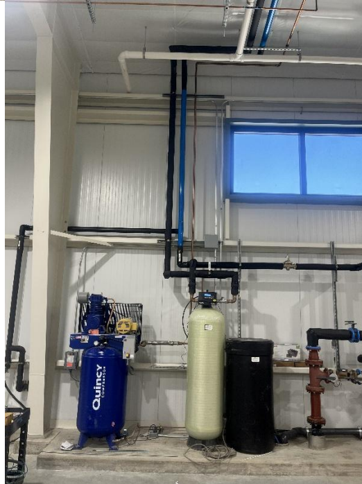
Non Potable Water system insulation installed.
