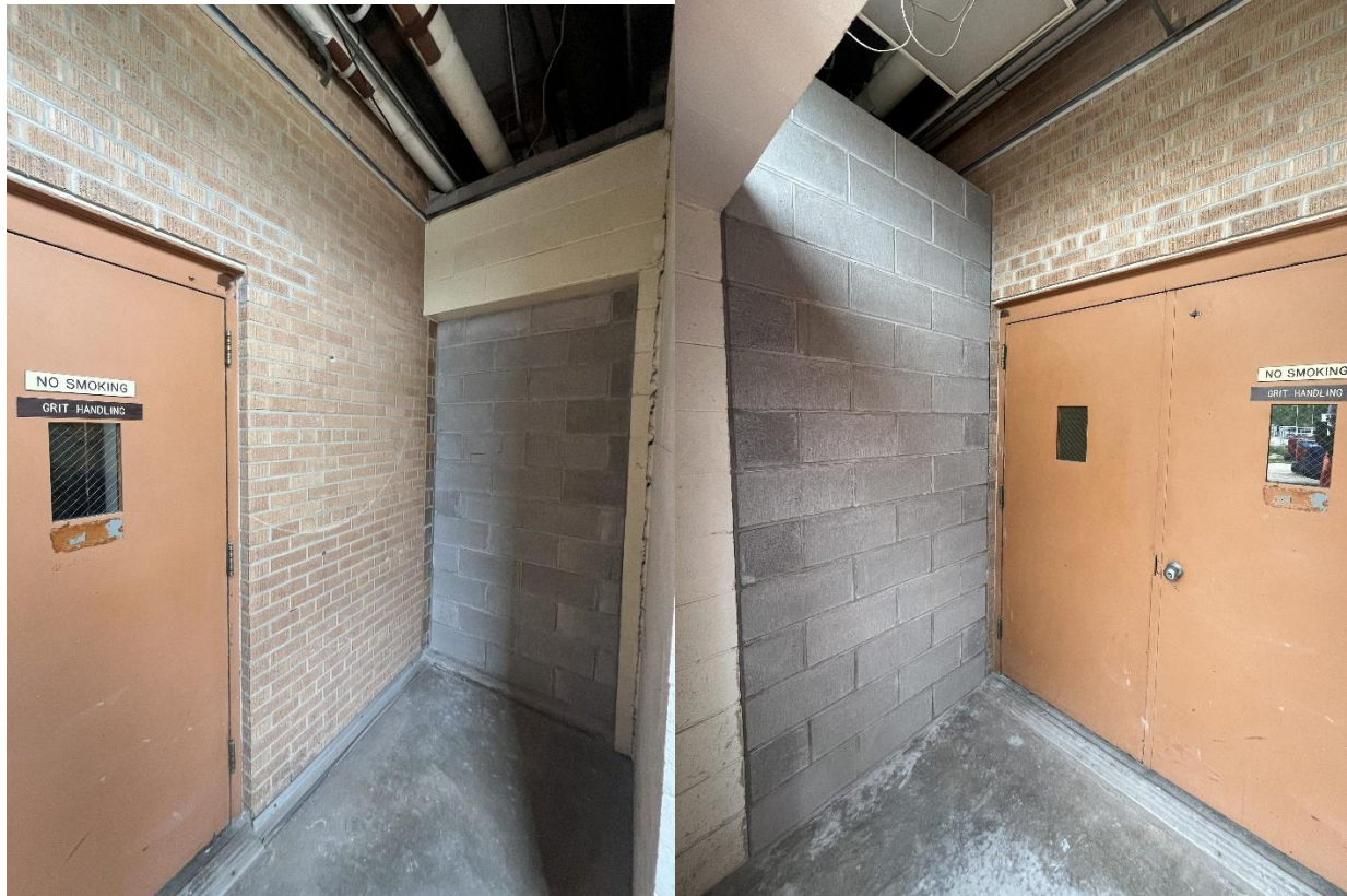
STR 100 bathroom and hallway CMU walls installed.
