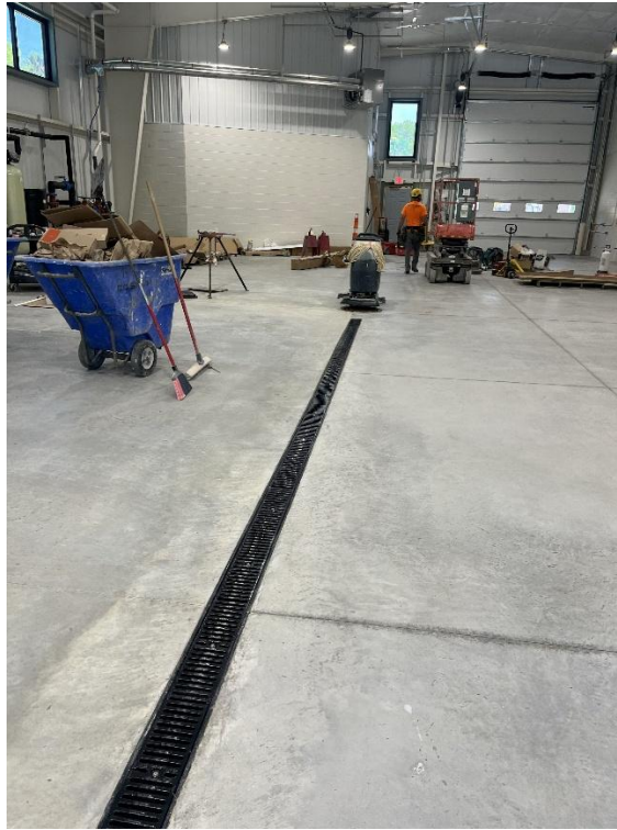
Garage floor sealed and trench grating installed.
