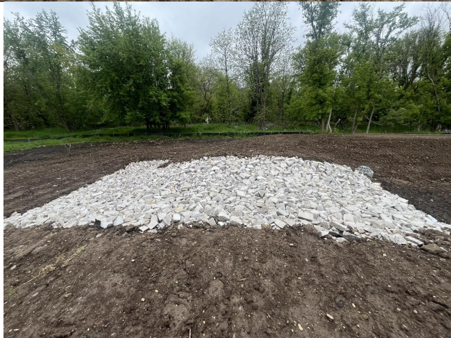
Overflow spillway lined and RIP RAP installed. STR 800 West Pond.
