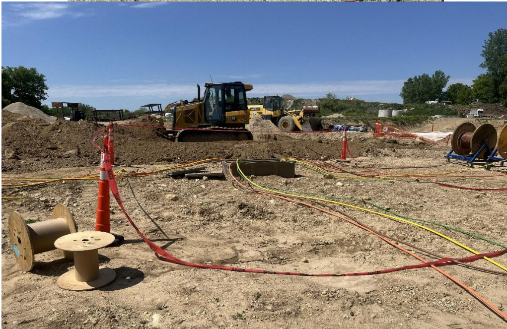
Electrical feeders being pulled across site from STR 800 to STR 100 & STR 650
