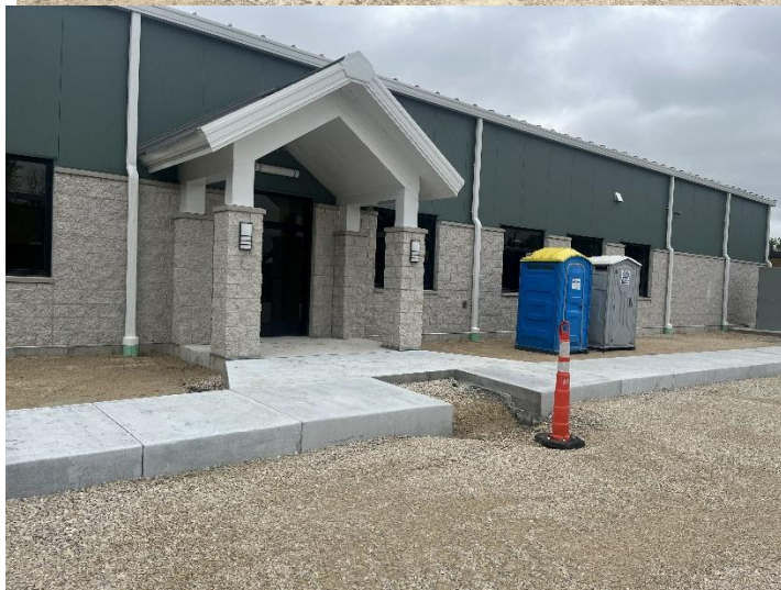
STR 800 / Site Concrete work continuing.
