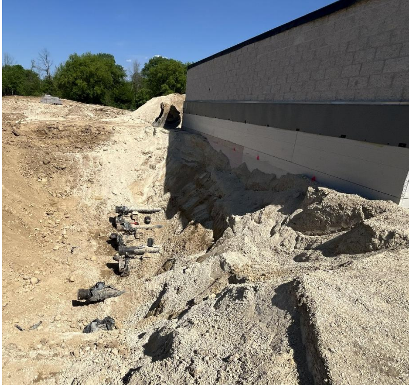
STR 600/650/700 underground piping and sludge manhole piping being installed.
