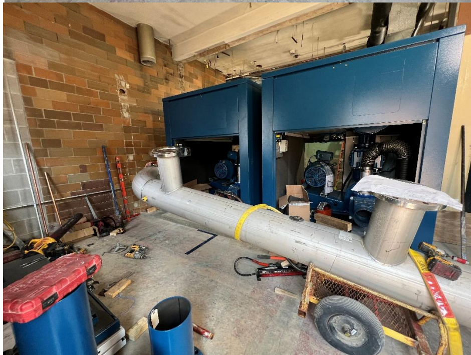
Blowers are set in place, STR 100.
