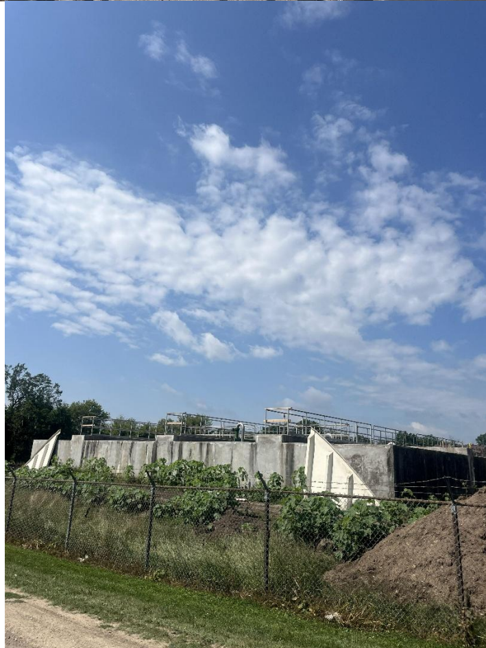
STR 200 cover removal complete.
