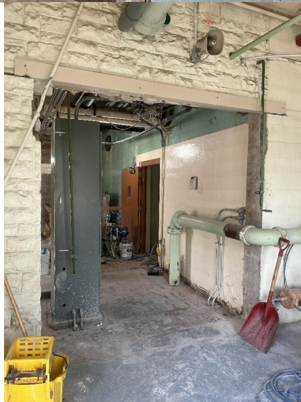
STR 100 hatch install, blower pad, and wall demo.
