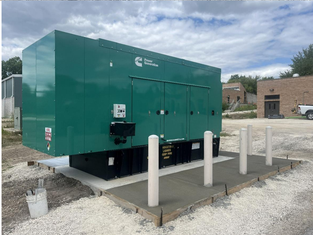
Site concrete around STR 650 and Generator.
