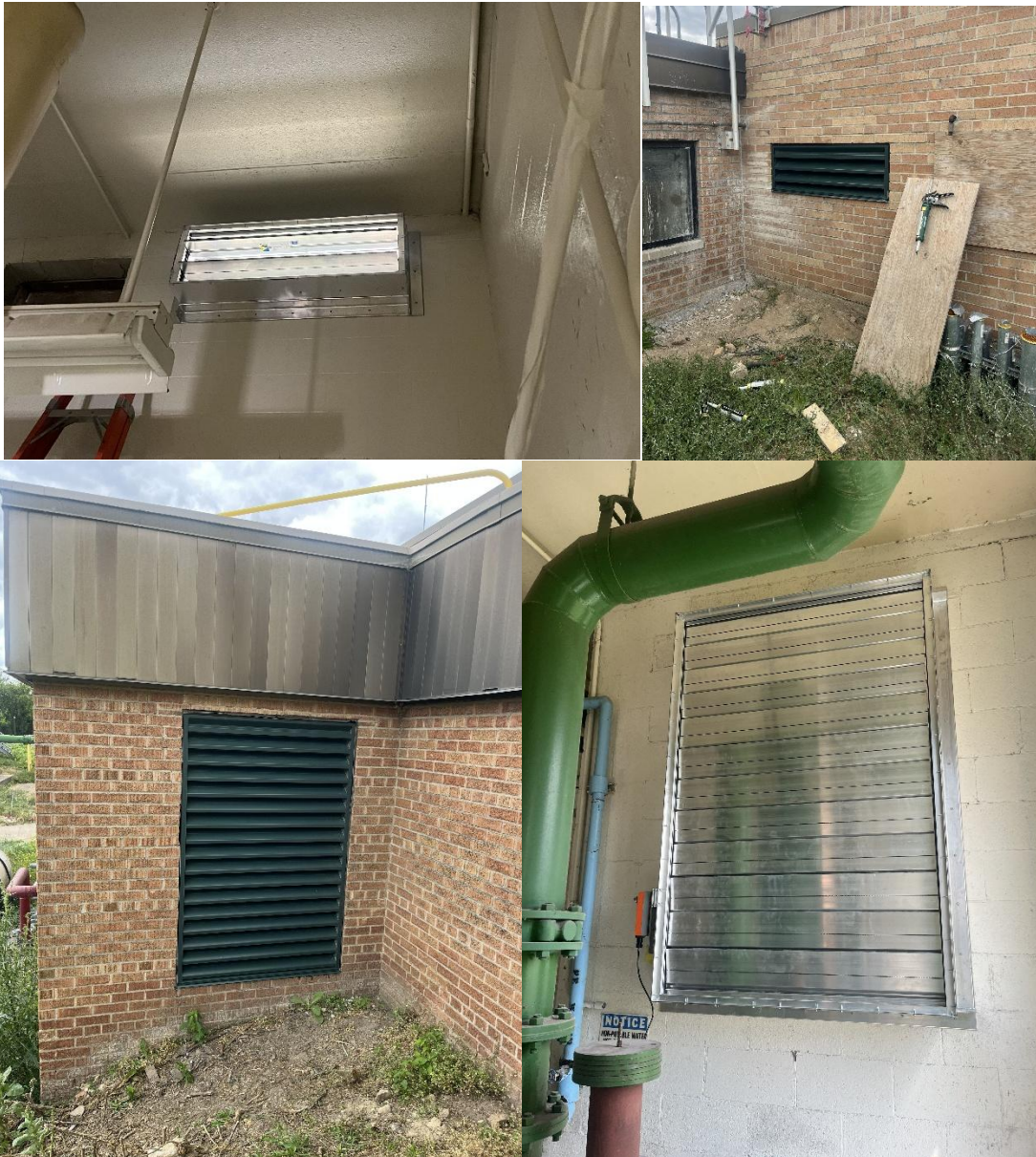
STR 100 Louver Installs.
