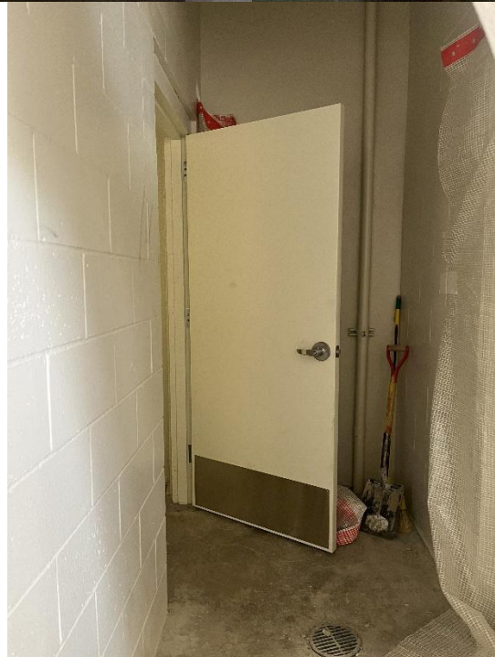
STR 100 Bathroom fixtures and door.
