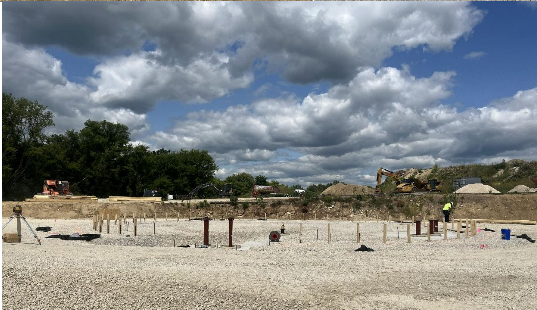
DN tanks mobilized to site. Prepping Wall forms.
