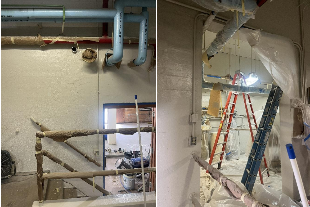
STR 100 Electrical and Mechanical Rooms painting.
