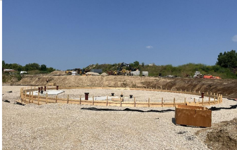
Wall forms prepped for STR 600 and 700. Rebar being installed on STR 600.
