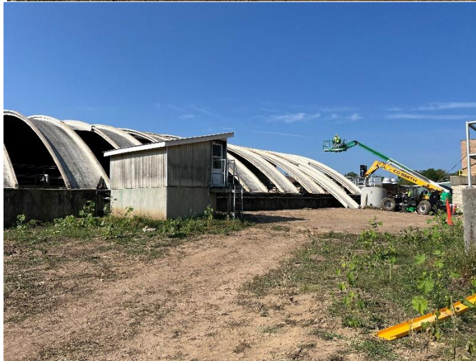
STR 200 Side wall removal and beginning of cover removal.
