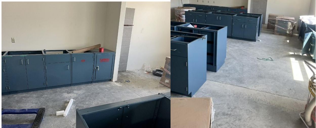
Laboratory cabinetry installation in progress.
