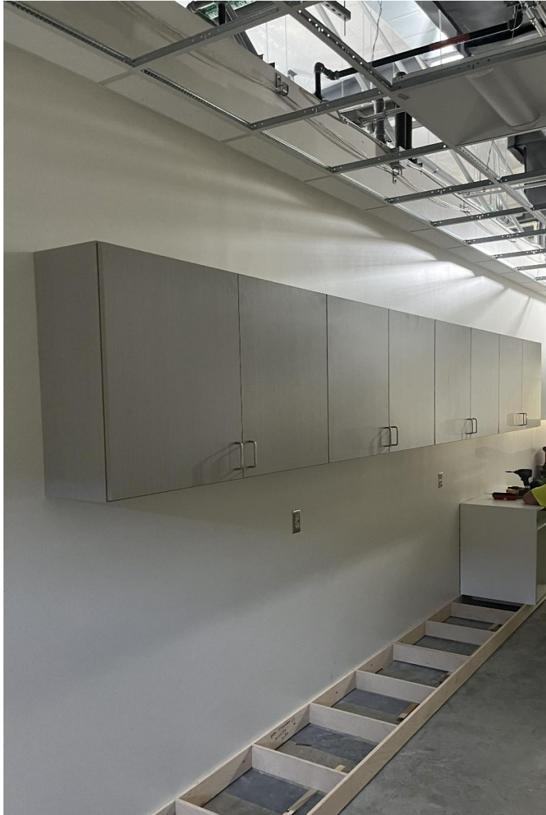
STR 800 hallway cabinetry being installed.
