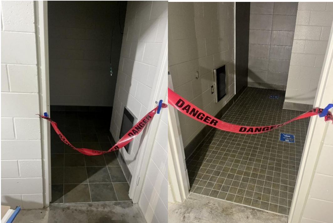
STR 800 shower and bathroom tiling being completed week of 4/20.
