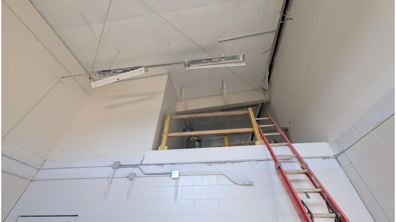
STR 800 workshop/mezzanine area during painting
