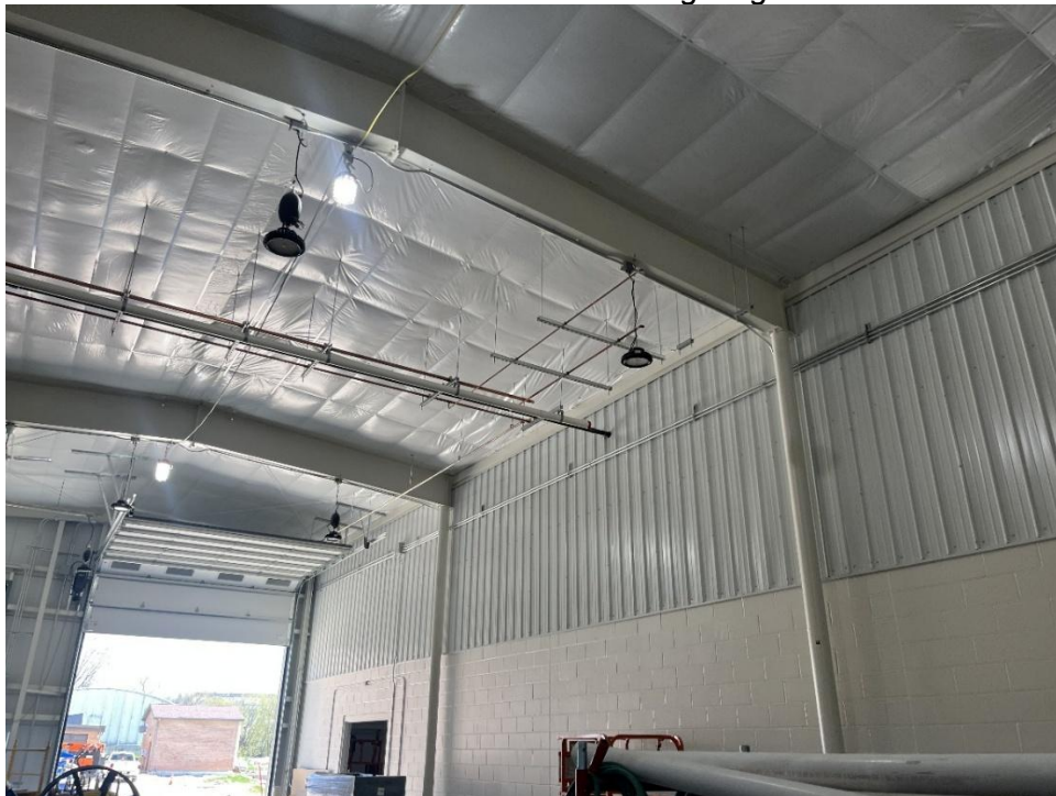
2-hour firewall finished and closed off to ceiling.
