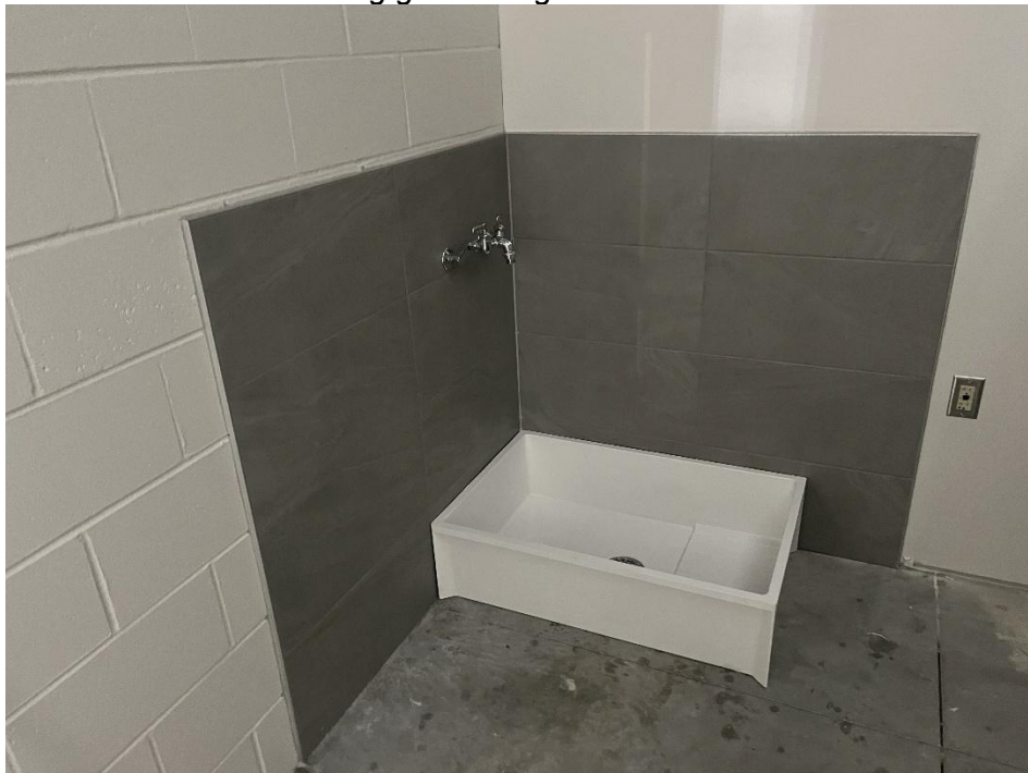
STR 800 janitors sink is installed.
