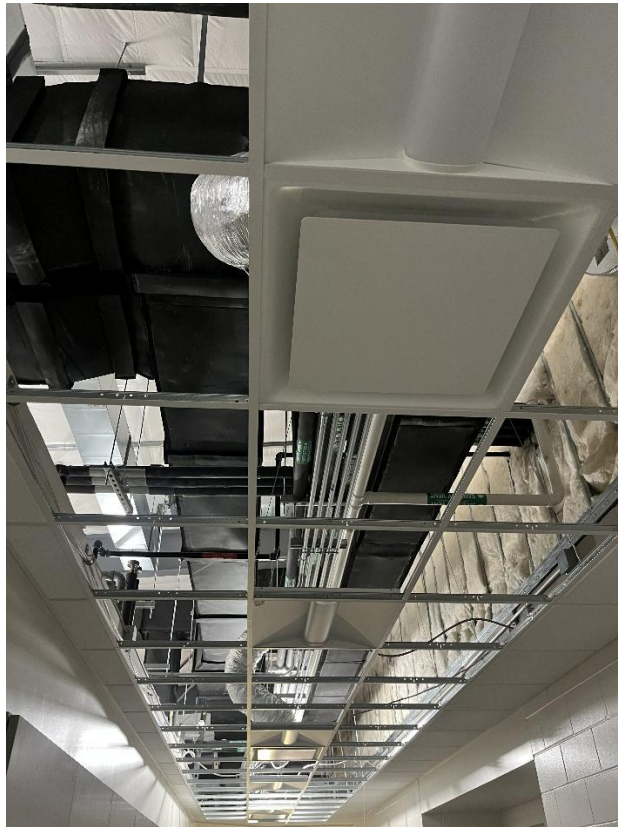
STR 800 ceiling grid and light fixtures are installed.
