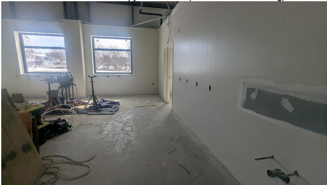
Laboratory walls painted, windows installed
