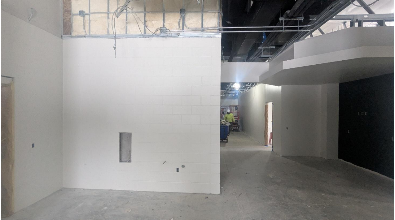
STR 800 breakroom area painted, teaming area ceiling installed/painted
