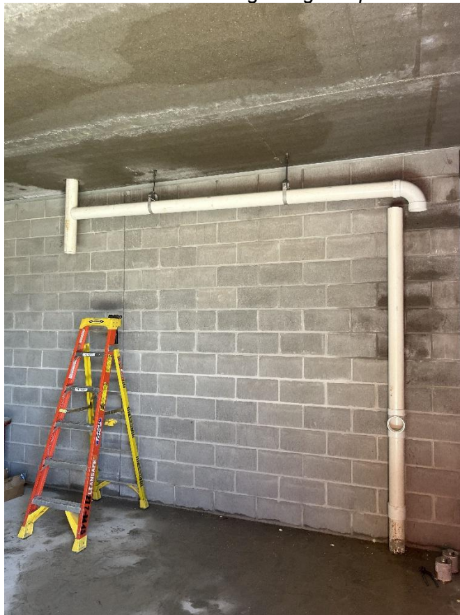
STR 650 Plumbing being installed.
