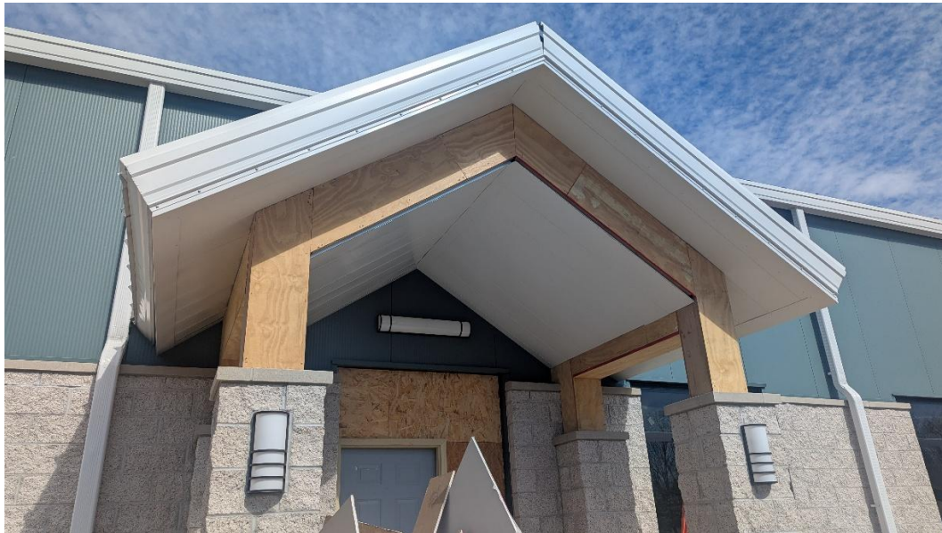
South entrance canopy of STR 800 (Administration building)
